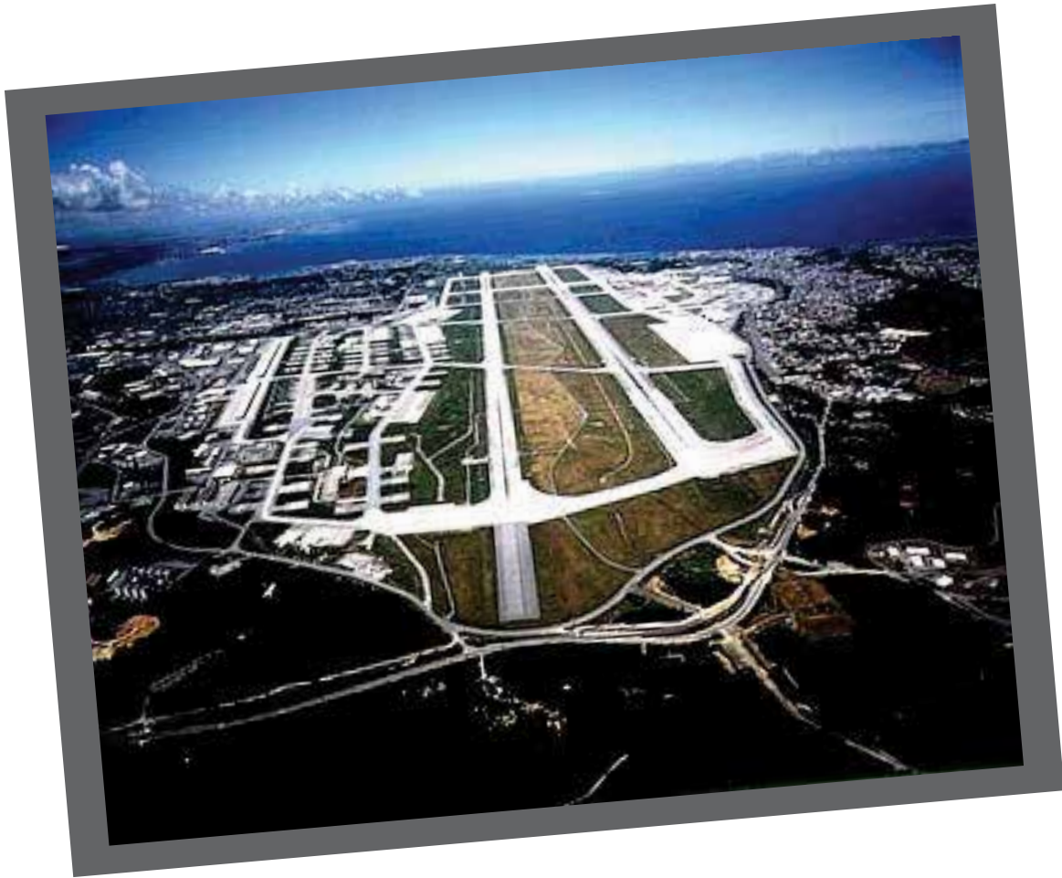
All of the OXCART's operational missions were flown out of Kadena Air Base on Okinawa, shown here.
